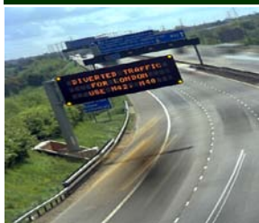
Kontrolni saobraćajni centar (Traffic Control Centre - TCC)
